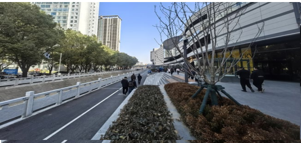
River Improvement at Nanyang High-Tech WUYUE Plaza
